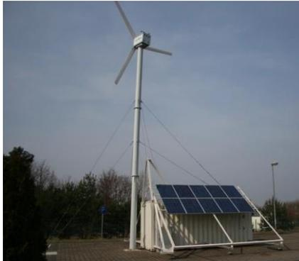
Off or on grid operation or a combination of the two is possible. The external dimensions of the sea container allow the operator to shift the power plant in one day to another location to start-up again.
