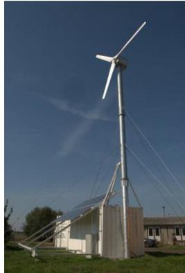
The JUWELIS Energy Container is a hybrid power plant that ensures the highest available of reliable energy without connection to an electrical grid.
